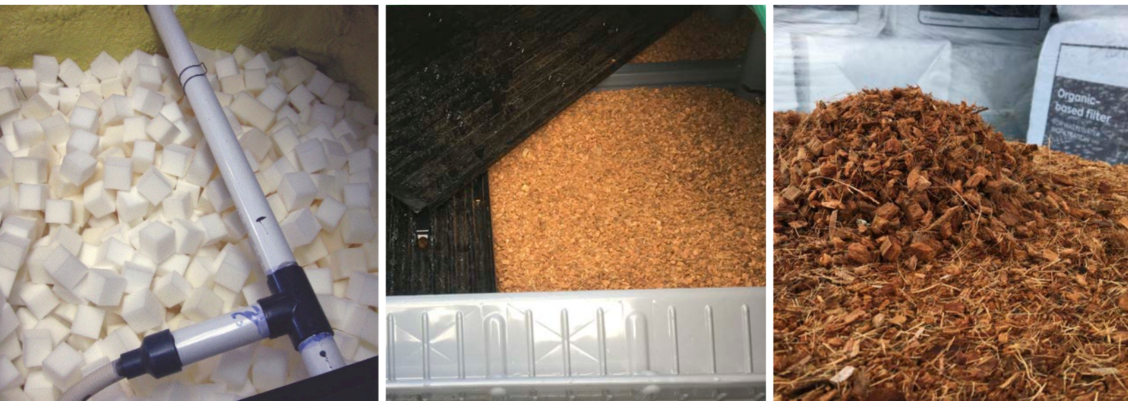
Effluent is distributed onto a synthetic media – foam cubes, peat moss or coconut fiber – for aerobic treatment.
